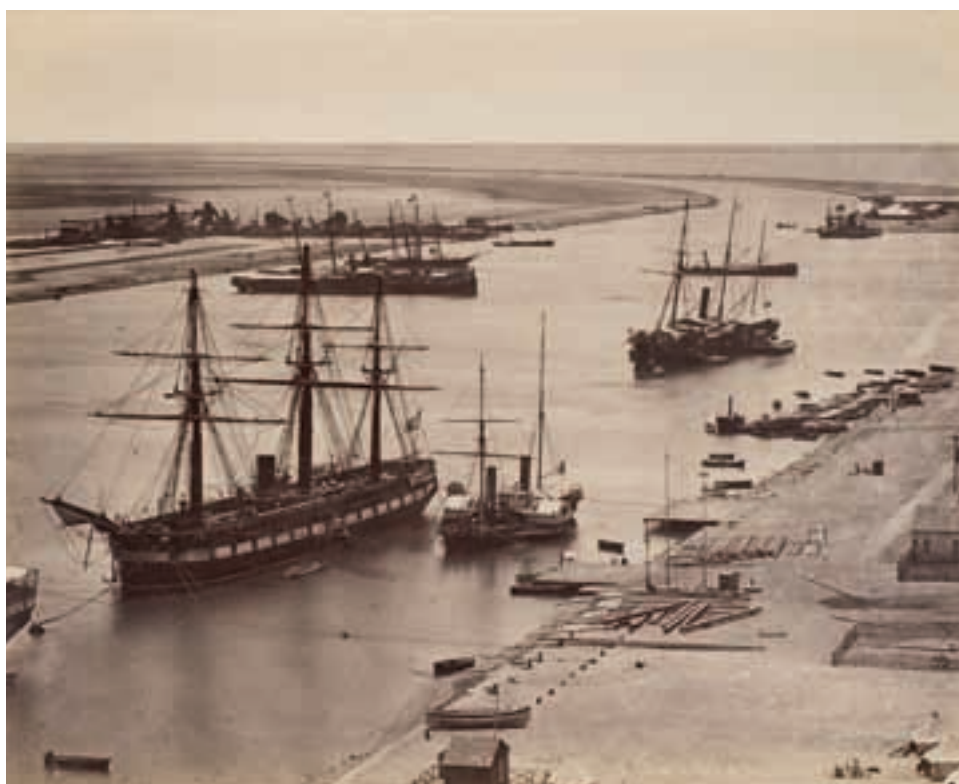
144 Vista parcial de Port Said.
