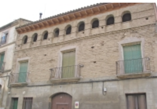
Binaced. Casa Laguna
